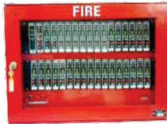
Conventional Fire Alarm Panel
